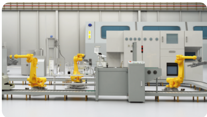
Safety Protection in Factory Work Areas
